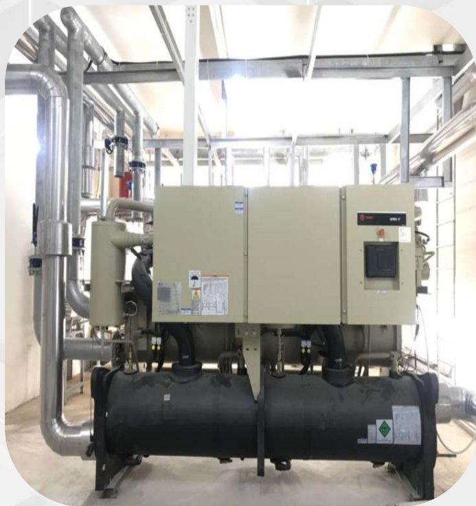
Chiller trục vít /Screw Chiller
