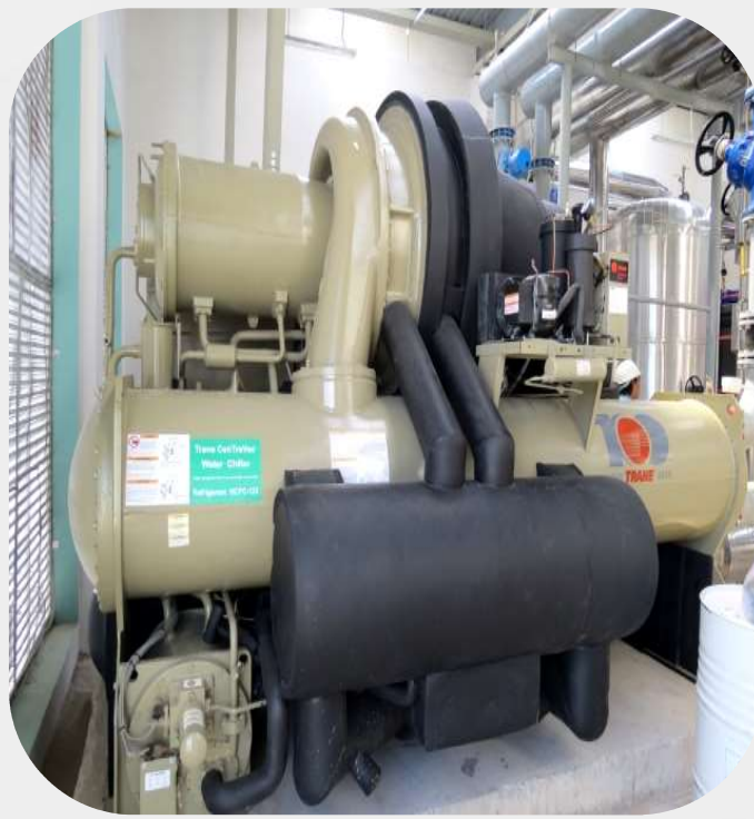
Chiller li tâm /Centrifugal Chiller
