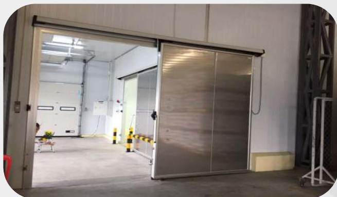
Cửa kho lạnh/Slide door for cooling room
